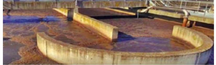
Removal of organic substances and nitrogen in treatment plants takes place mainly through **biological oxidation in aerated tanks**. Since in a conventional activated-sludge plant the **energy demand is largely due to aeration**, attention has focused on the development of new technologies for reducing the energy consumed for the transfer of oxygen.
